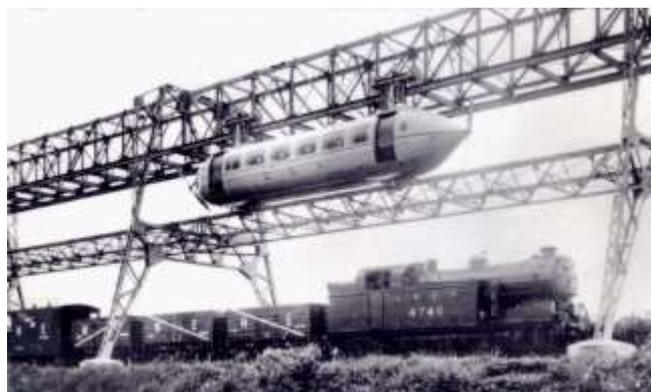
near Glasgow was the Bennie rail plane, (picture) designed to travel above existing rail lines at 150 mph using an
